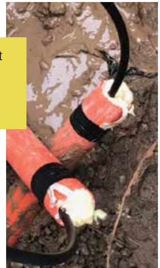
Figure 3. Foam makes a great temporary seal so segmented conduits can be easily accessed in the future.
