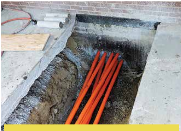
Figure 2. Segmented conduits are installed in the same manner as standard HDPE conduits.
