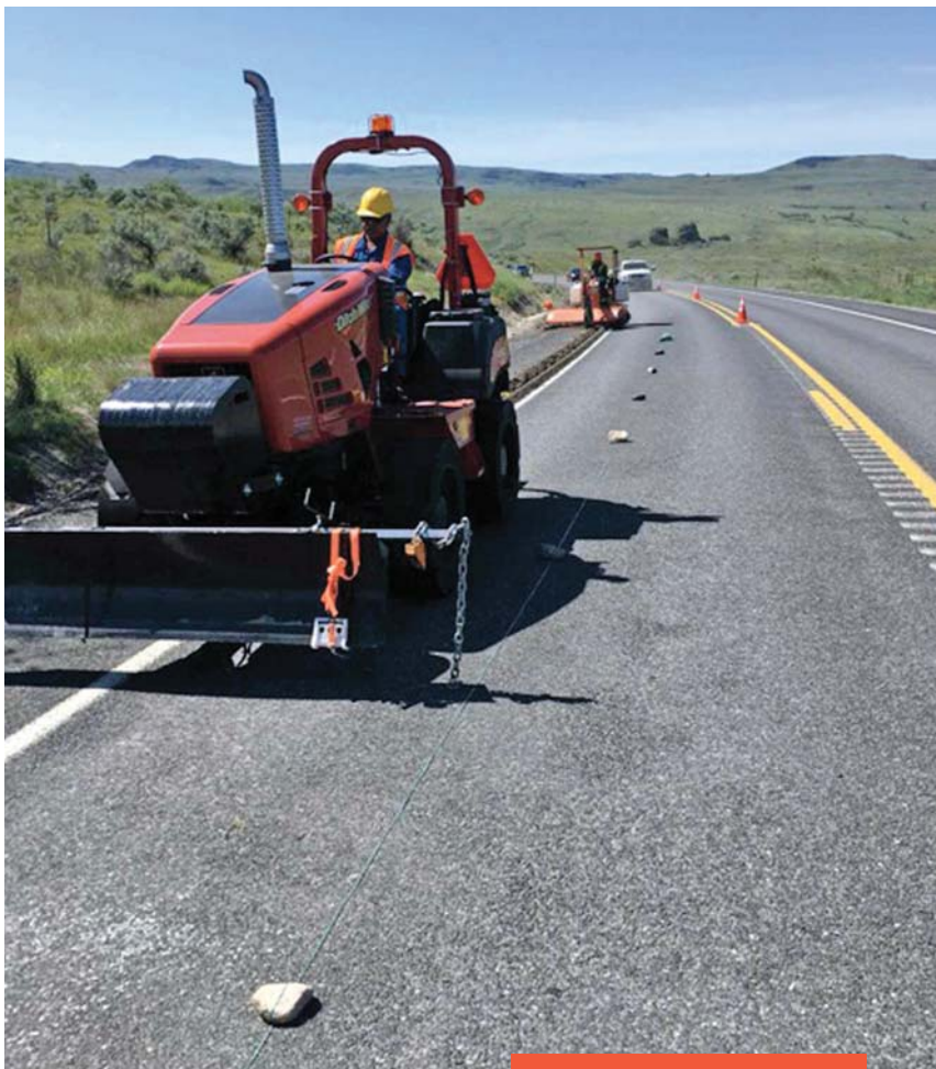
Figure 3. Microtrenching in rural British Columbia, Canada.
